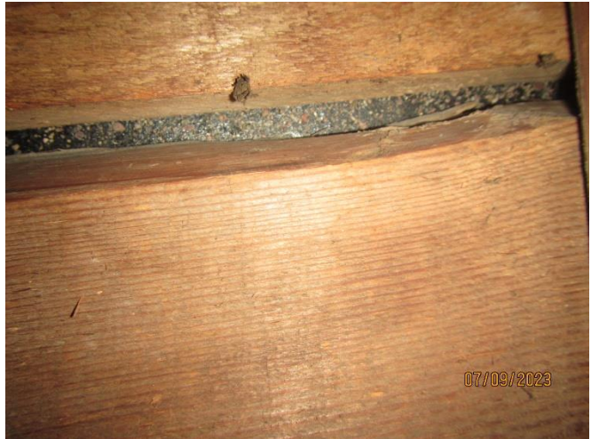
Bitumenfilt under plåttaket.
